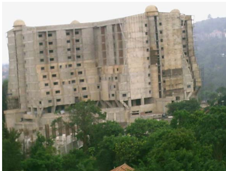
Construction work in progress
