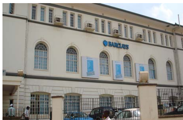
A bank in Kampala
